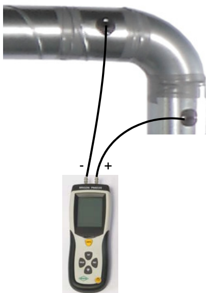
Fig. 3.22 Measuring the differential pressure with the digital manometer
